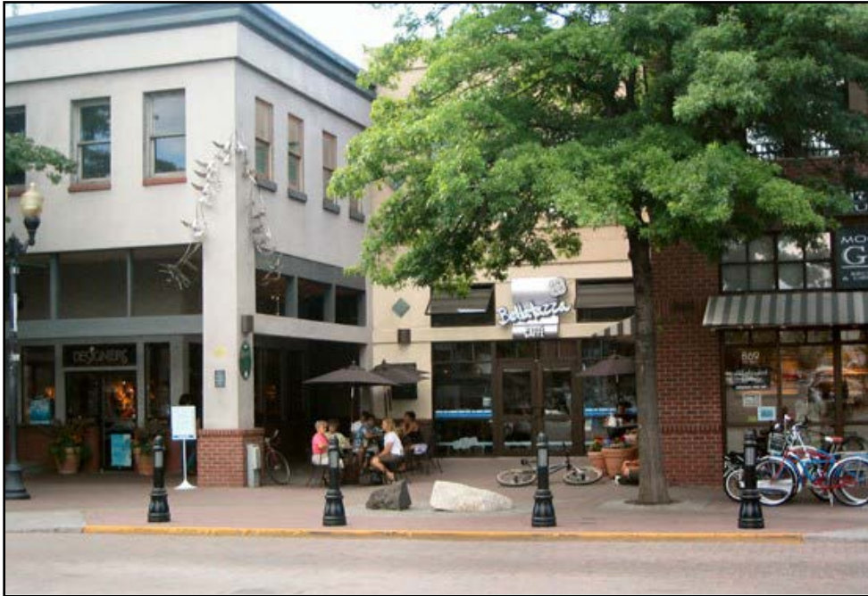
Figure 3-13 Typical Retail Building
