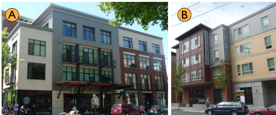
Figure 25.71.460.B Acceptable metal siding examples.
