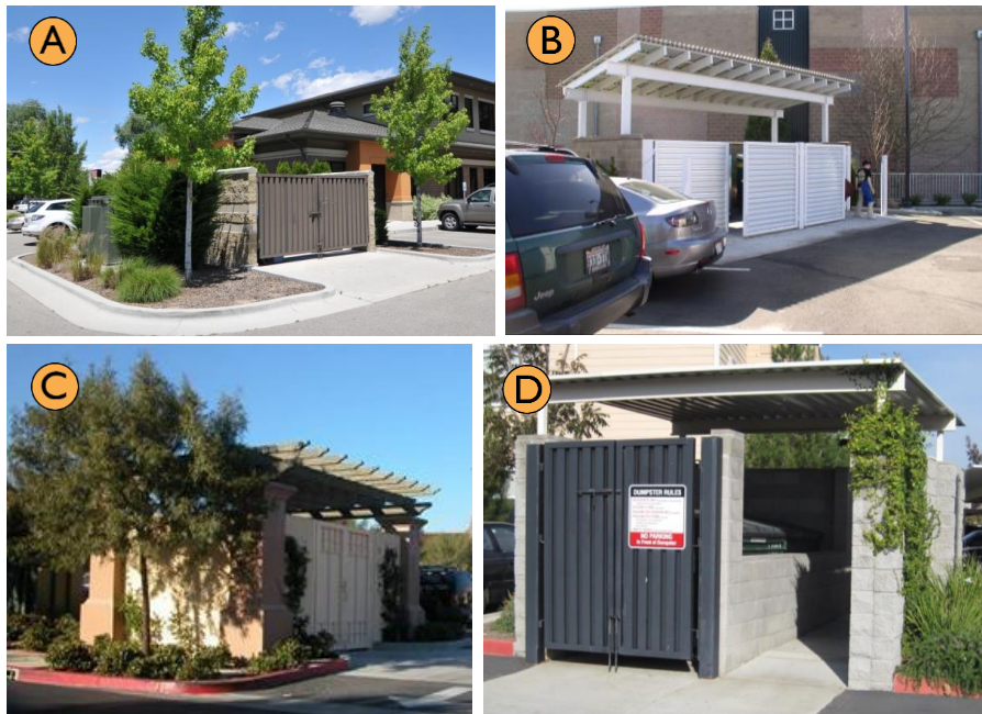
Figure 25.71.320.J Acceptable trash screening enclosures.
