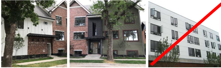
Figure 25.71.460.C Acceptable and unacceptable cementitious wall board examples.
