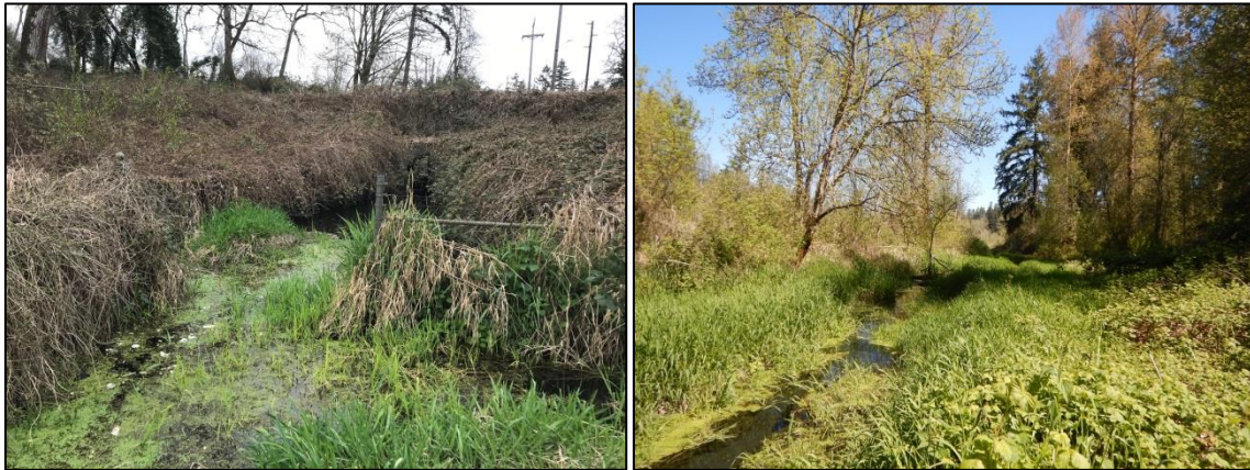
Figure 2. Stormwater Outfall and Channelization
