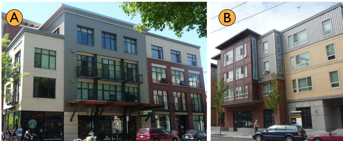
Figure 25.71.460.B Acceptable metal siding examples.
