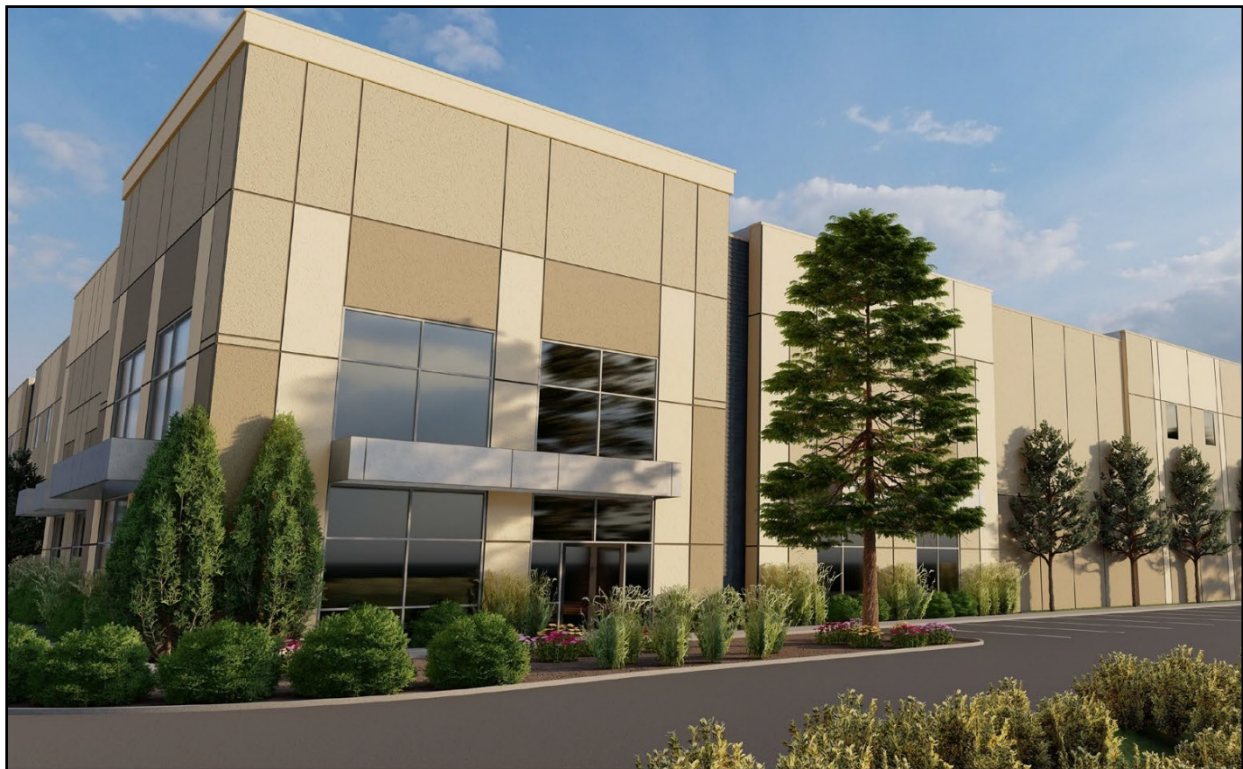
Figure 3-9 Typical Manufacturing Building
