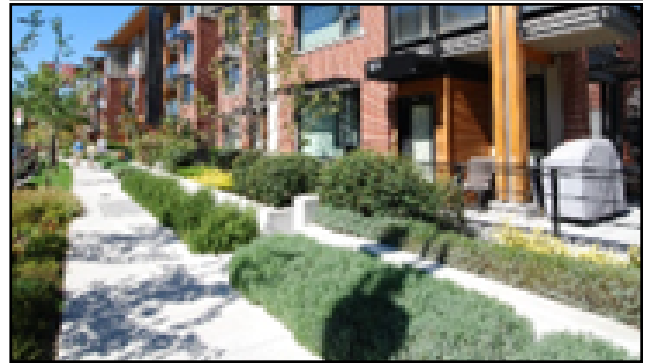
Figure 10 - Multifamily buildings with stoops and terraced planters.
