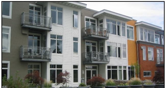
Figure 3 - Example of a multi-tenant commercial building with roofline changes, weather protection, and vertical building modulation.
